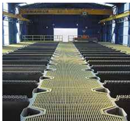
Detalle Nave EW.
